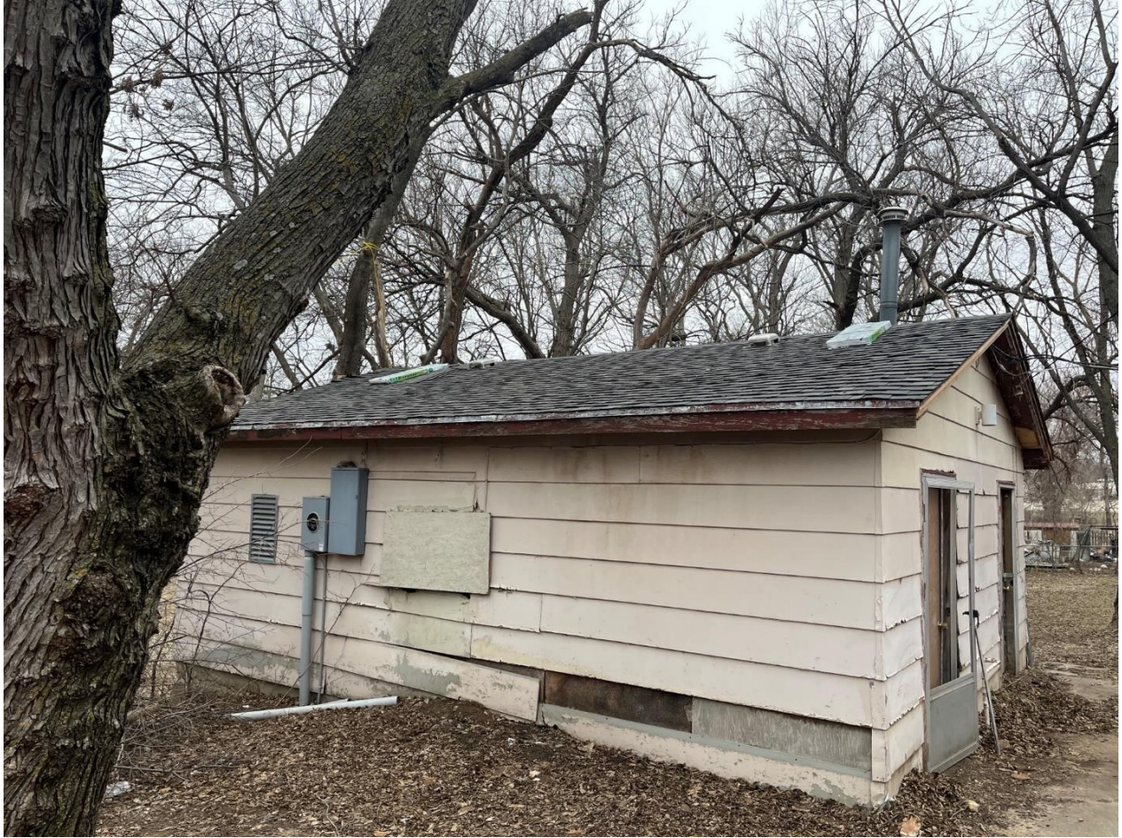
Photos Taken 2/4/2025 (Shed in Back)
