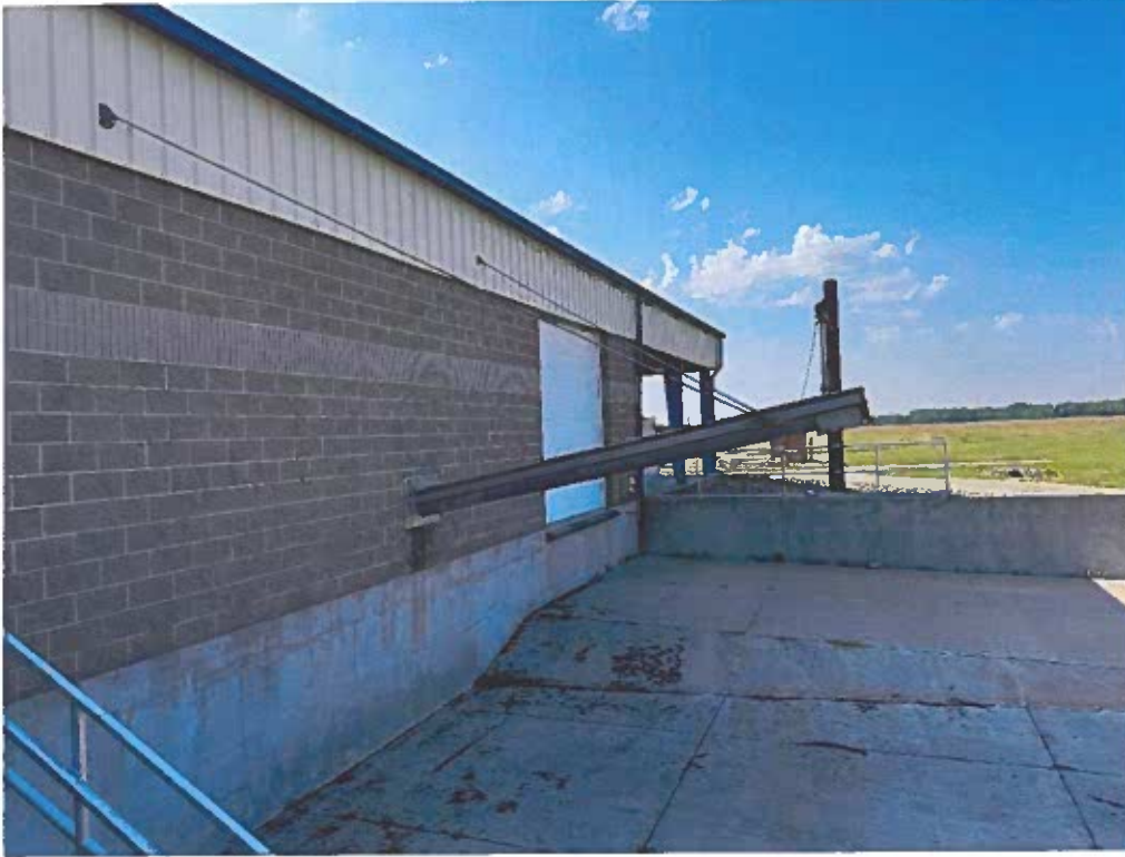
Figure 7: South end of west elevation.
