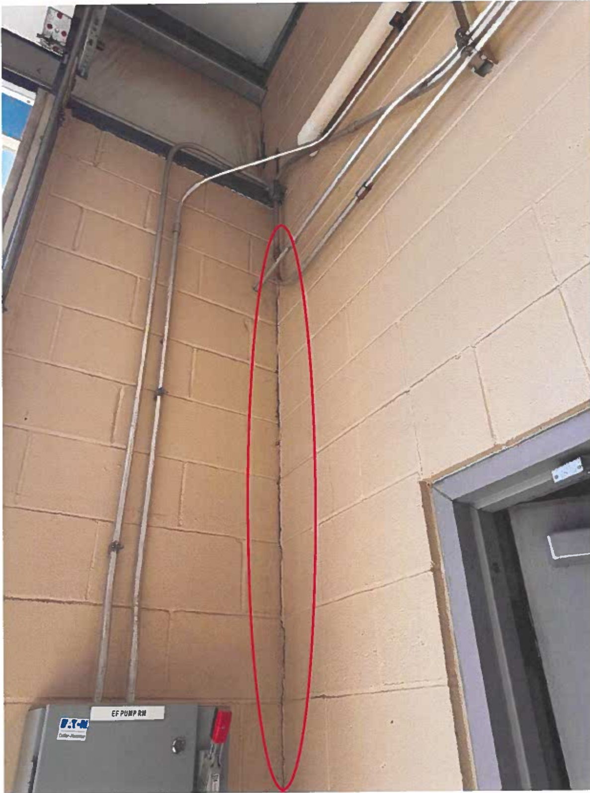
Figure 12. Note rigid frame cast tightly in masonry wall.
