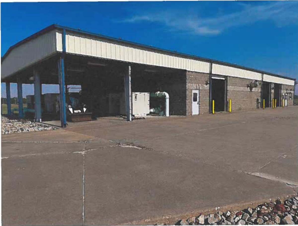
Figure 1: Process Building east elevation.
