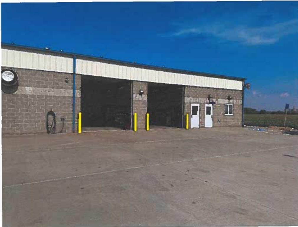
Figure 4: North end of east elevation.
