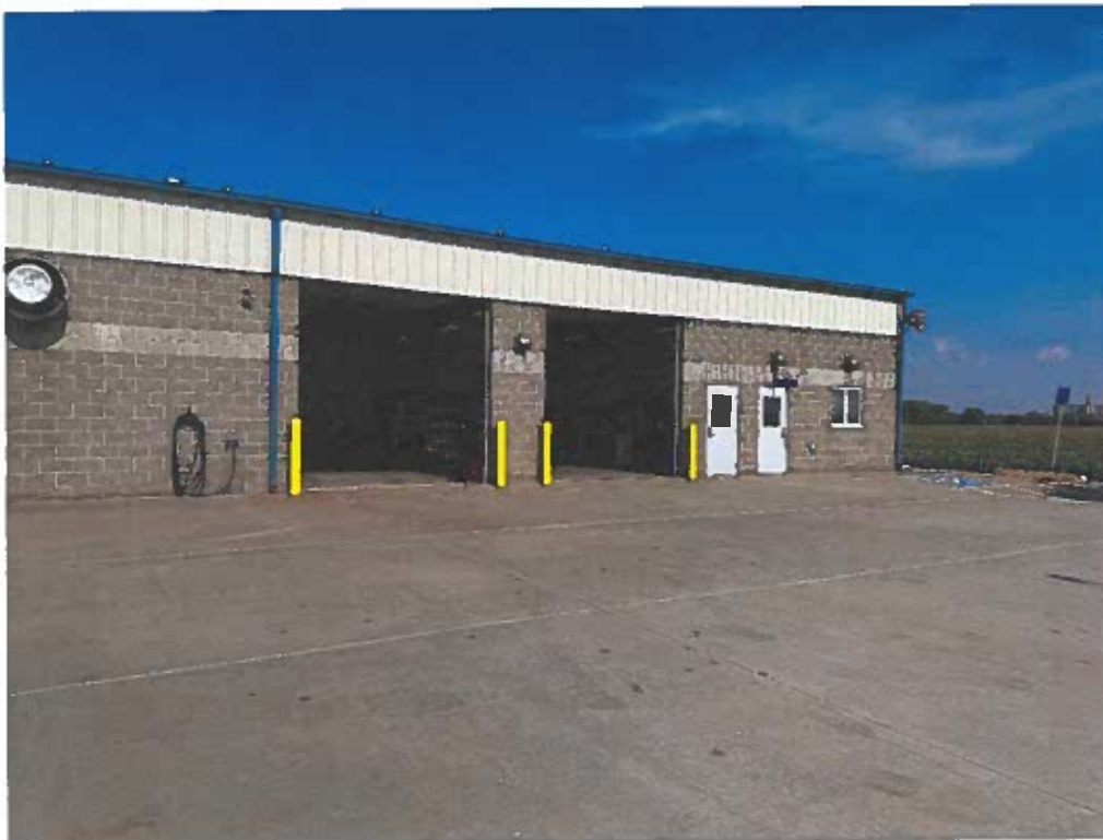
Figure 4: North end of east elevation.
