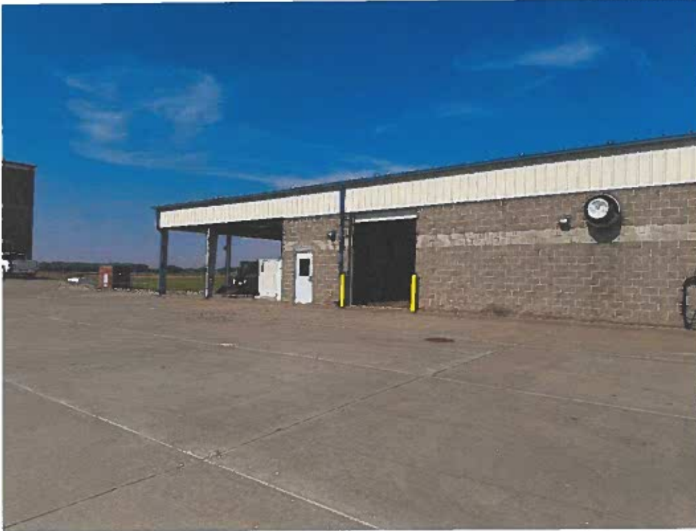
Figure 3: South end of east elevation.
