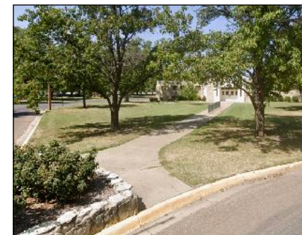
Concrete sidewalk at Municipal Pool entrance
