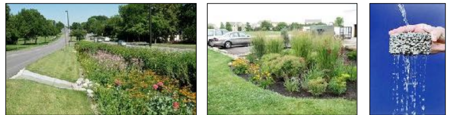
Bioswale, raingarden & permeable concrete
