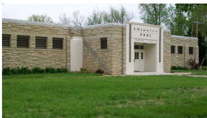
Bathhouse south elevation. Photo by William E. Fischer, Jr., 5/1/2011
