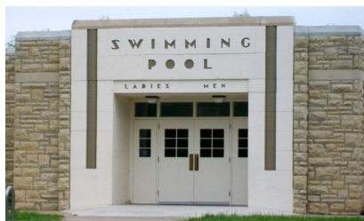
Bathhouse south elevation, main entrance detail. Photo by William E.
