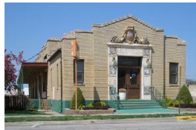
Union Pacific Freight Warehouse
