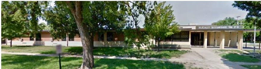
McKinley Elementary School
