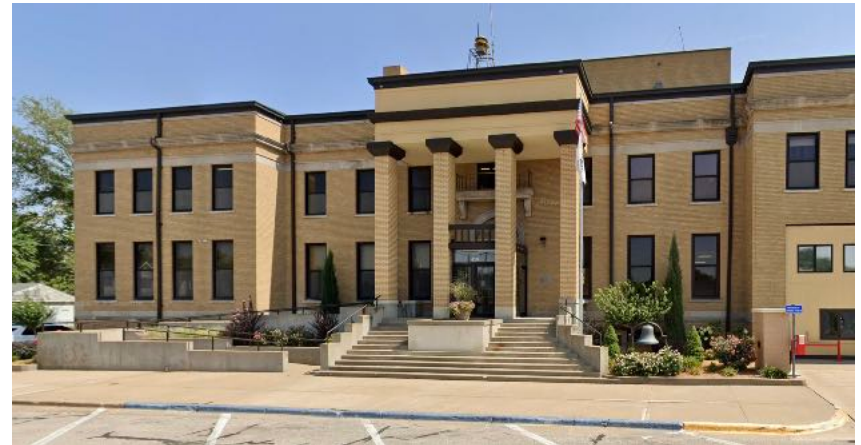
Abilene City Hall—west facade
