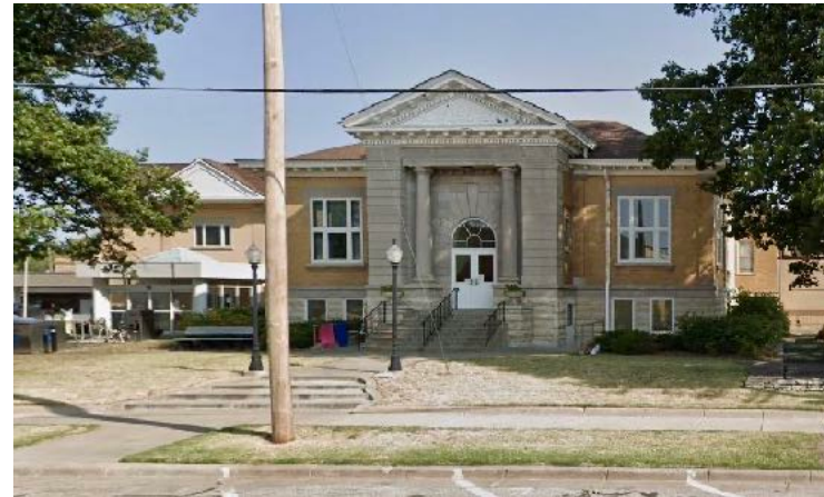
Abilene Public Library— south facade
