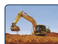
Construction Phase Services
