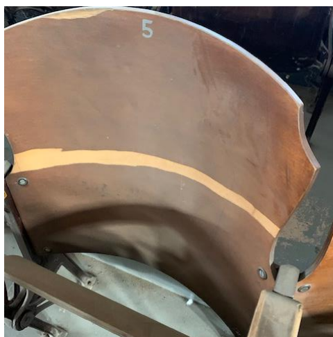
Damaged Wood Veneer
