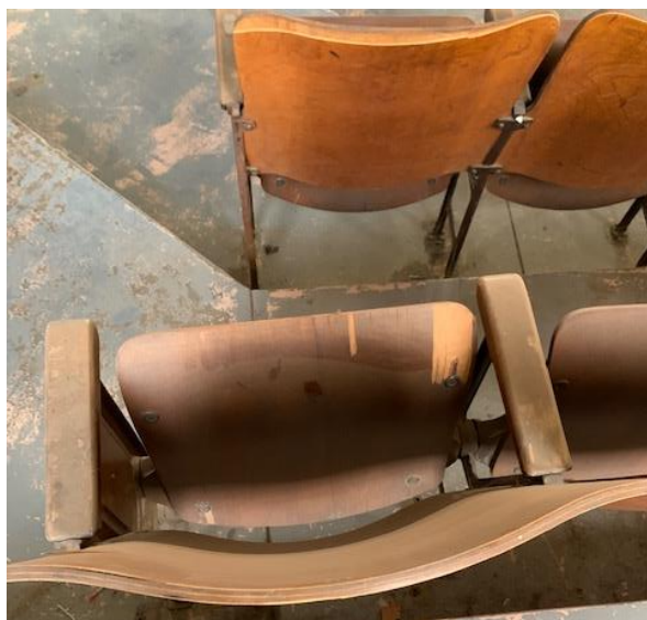
Damaged Wood Veneer
