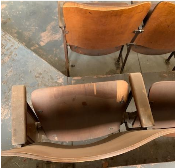
Damaged Wood Veneer
